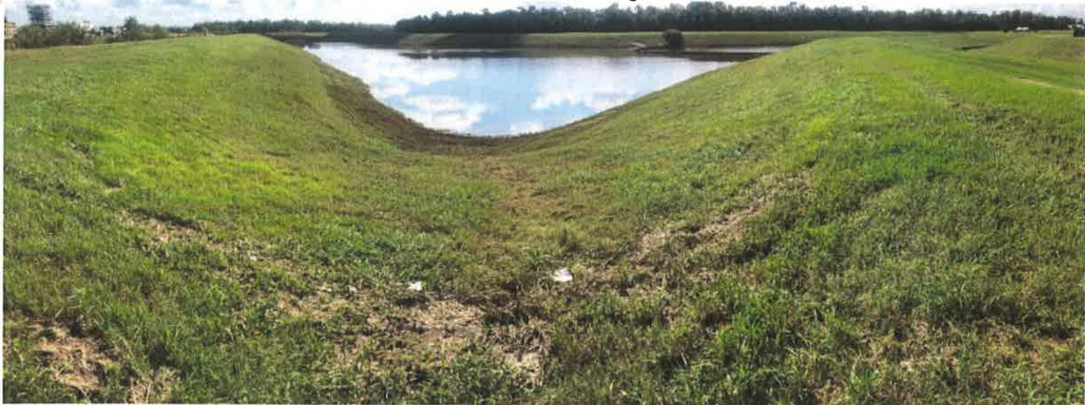
Southwest Corner of Pond Looking North & West
