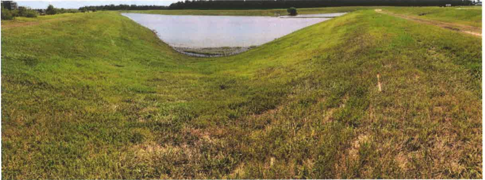
Southwest Corner of Pond Looking North & West
