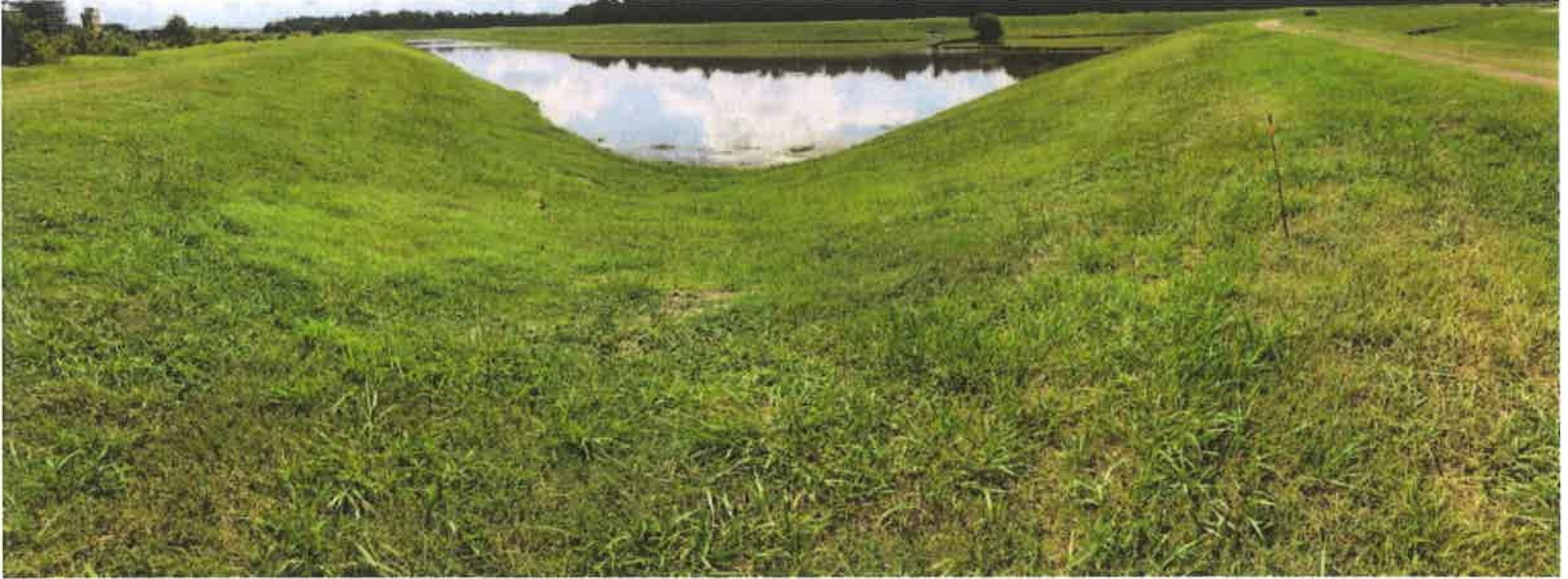
Southwest Corner of Pond Looking North & West
