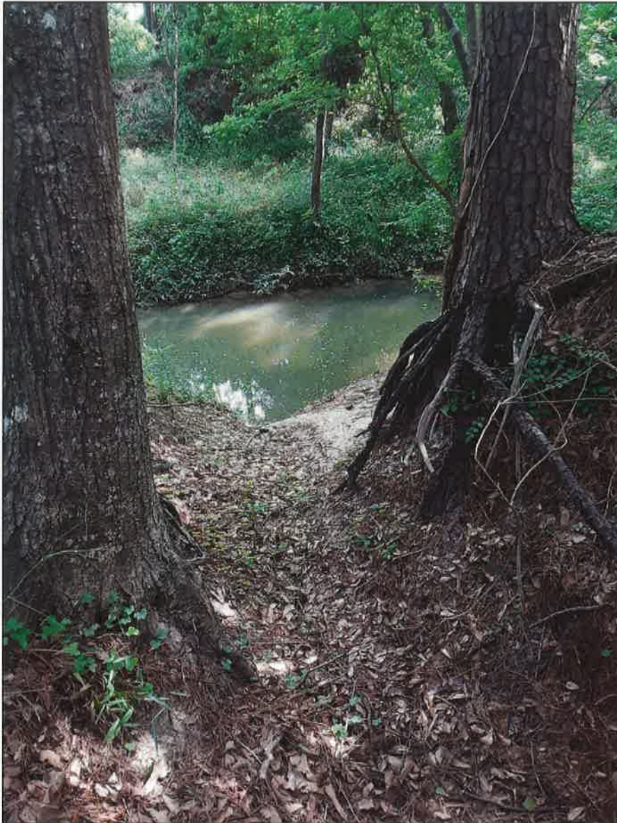
Photograph 4: View of Section C from south bank facing north bank showing erosional gully emptying into stream.
