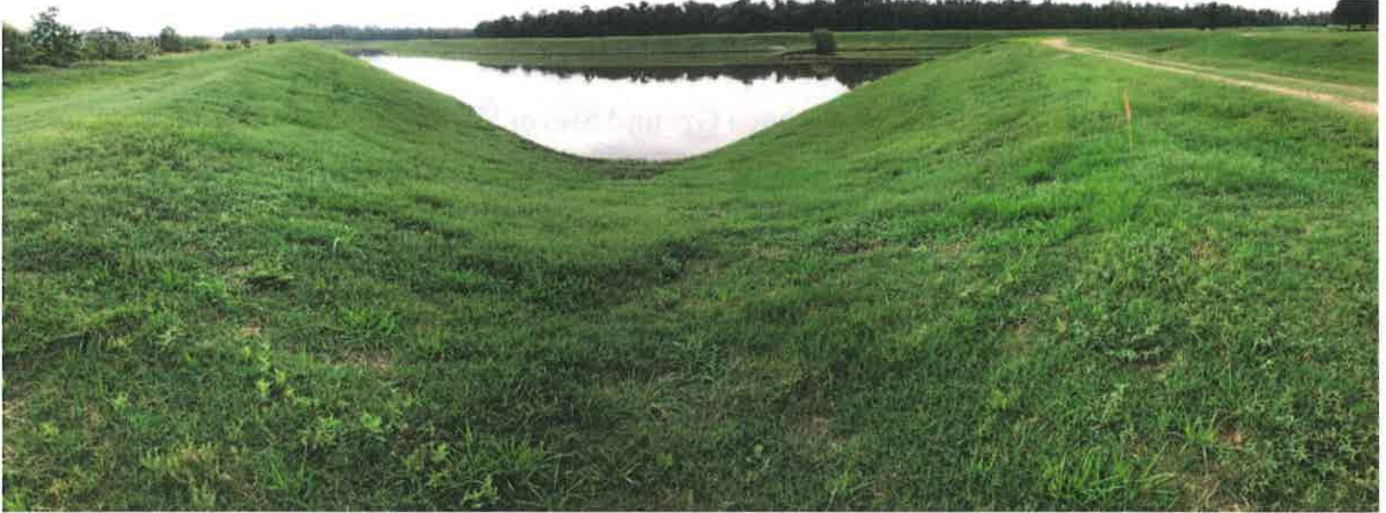
Southwest Corner of Pond Looking North & West
