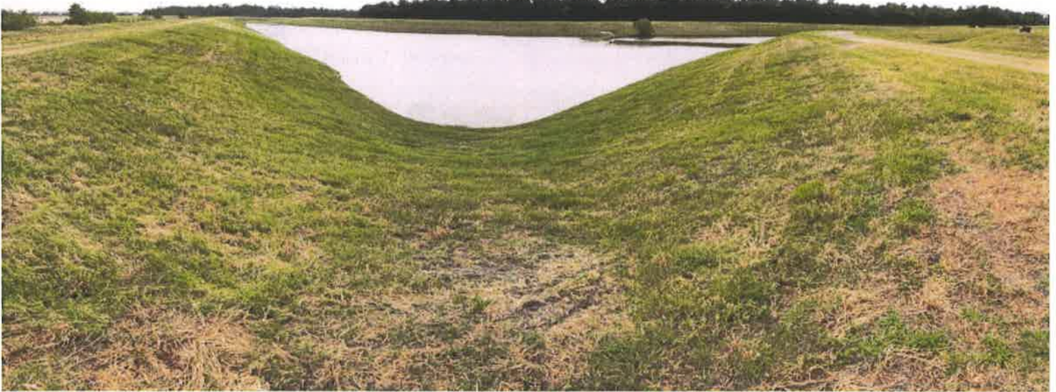
Southwest Corner of Pond Looking North & West
