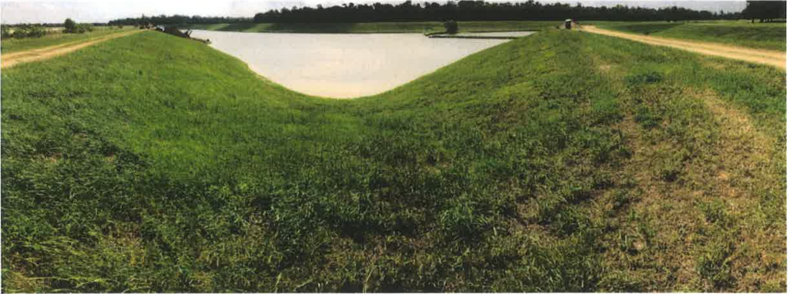
Southwest Corner of Pond Looking North & West
