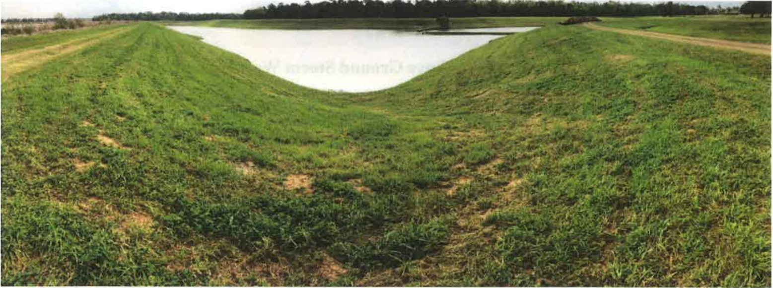
Southwest Corner of Pond Looking North & West
