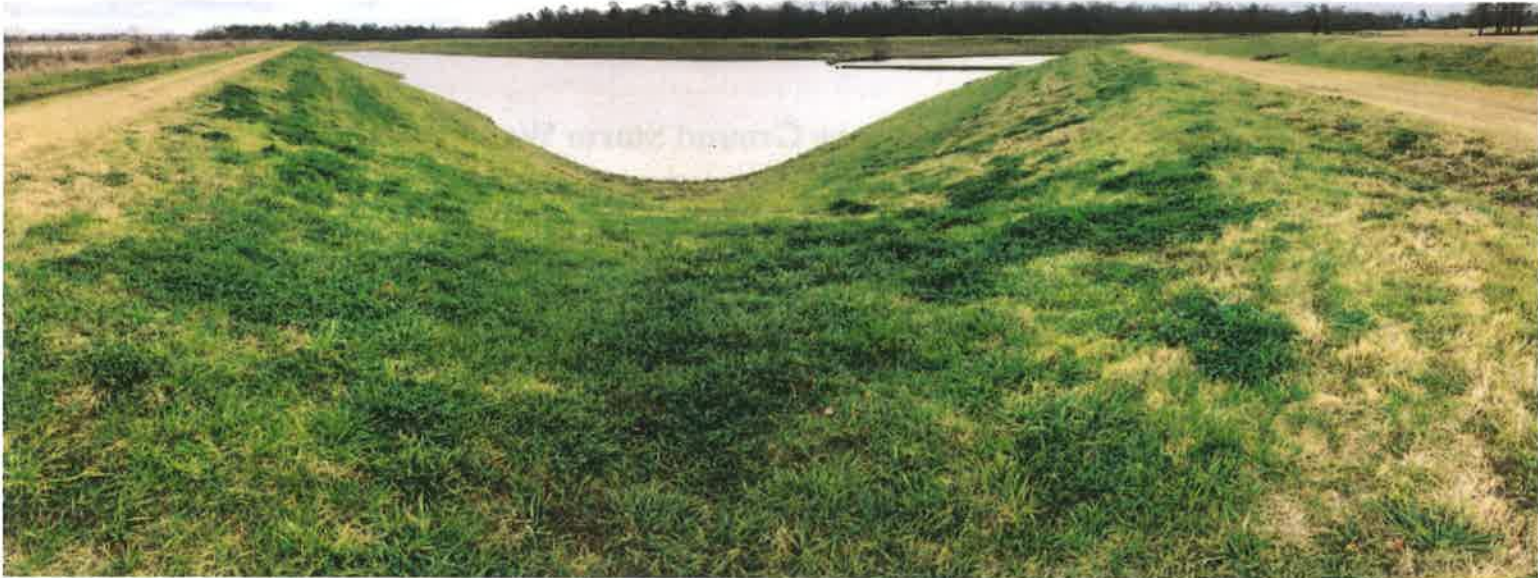
Southwest Corner of Pond Looking North & West
