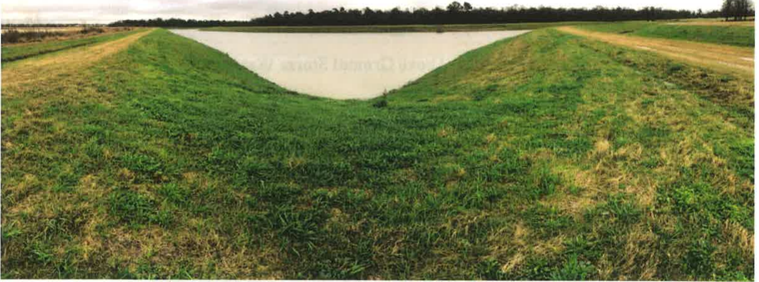
Southwest Corner of Pond Looking North & West
