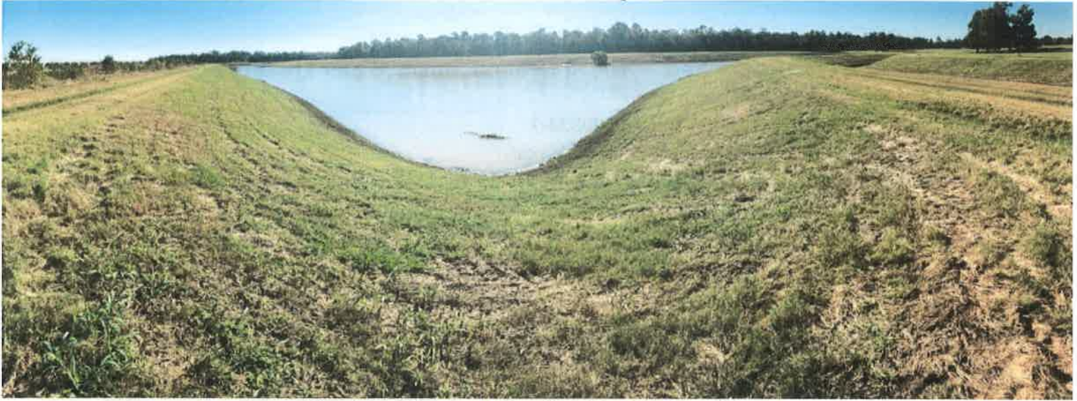
Southwest Corner of Pond Looking North & West
