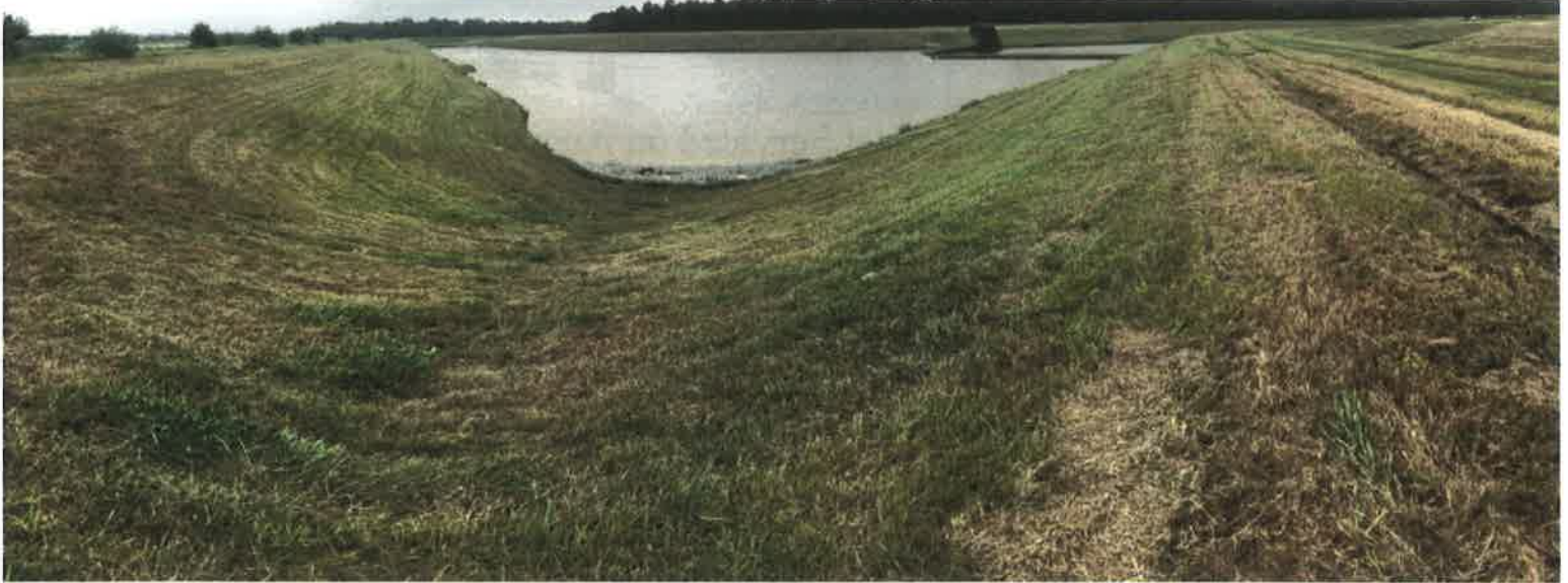
Southwest Corner of Pond Looking North & West
